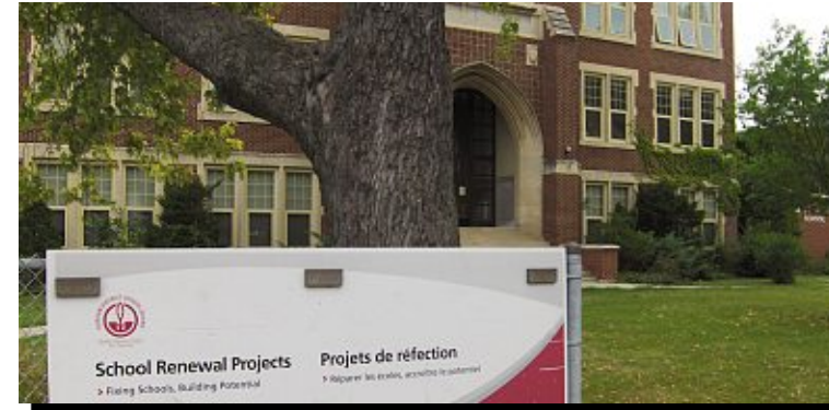
Oshawa Schools Renovation Project
