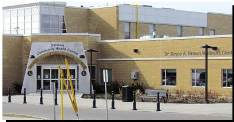
New Oshawa Community Health Centre at Conant Complex
